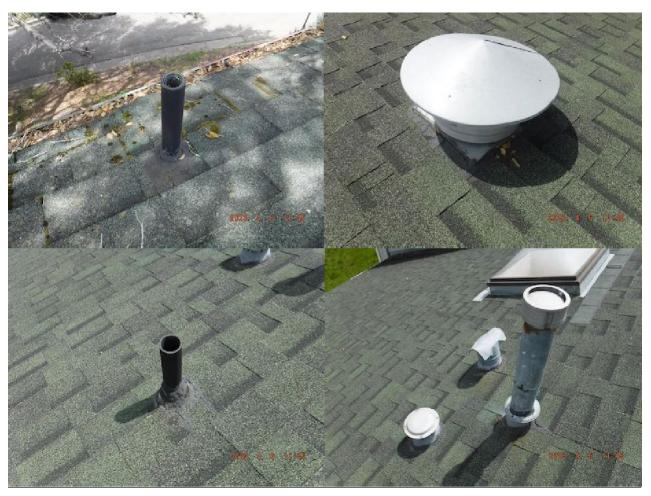
There are several unpainted black ABS (acrylonitrile-butadiene-styrene, the chemical make-up of a black plastic-composite plumbing pipe used extensively for drain, waste and vent systems) plastic plumbing vent pipes that are exposed to the sun. All exposed plastic pipes should be painted for solar protection.
