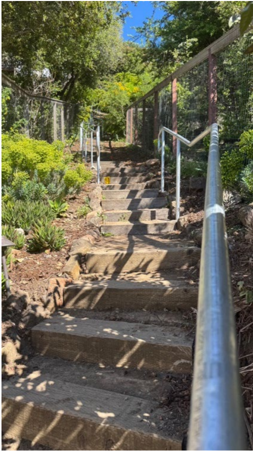
Beloit Path steps: New handrails on one side of all steps.
