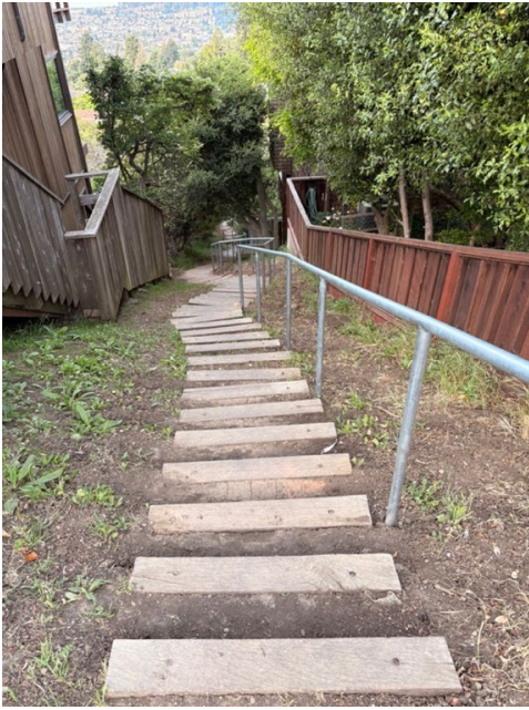
Beloit Path: Wood steps cleared of dirt and weeds with new handrail.
