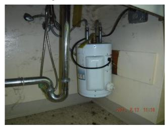
There was no hot water at the time of our inspection. The water heater was plugged into an operating electrical outlet and so is likely to have failed.
