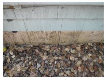
This condition can trap moisture in the wood and is conducive to decay. We recommend adequate clearance be provided as needed to eliminate embedded conditions.
