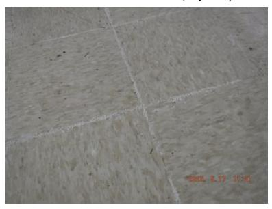
We recommend these floors be removed and replaced after the flooring has been inspected and suitably sealed using a properly rated sealant. Sealants should be selected, in part, based on what is to be installed over them. A good choice for replacement may be vinyl plank, if this is compatible with future anticipated use of the space. (e.g. This would not be a good choice if very hot items may be dropped or fall in the space as in glass blowing, ceramics, etc.)
