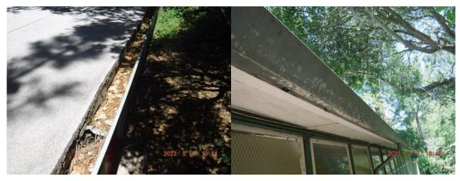
Several downspouts are damaged. See one below. We recommend all of the downspouts be replaced.
