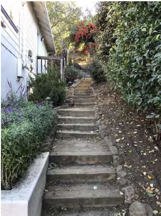
Beloit lower - Before Handrail
