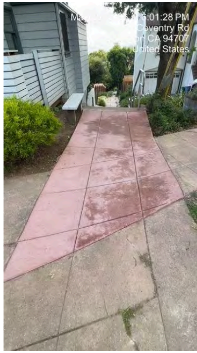
Coventry - New Concrete
