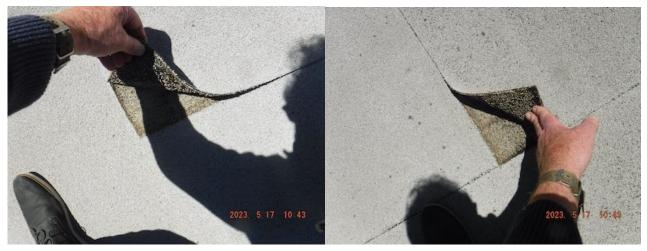
This may be an adhesive type of modified bitumen and normal without the typical adhering bead resulting for adequate heating.
