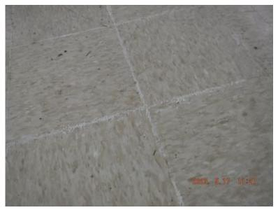
We recommend these floors be removed and replaced after the flooring has been inspected and suitably sealed using a properly rated sealant. Sealants should be selected, in part, based on what is to be installed over them. A good choice for replacement may be vinyl plank, if this is compatible with future anticipated use of the space. (e.g. This would not be a good choice if very hot items may be dropped or fall in the space as in glass blowing, ceramics, etc.)
