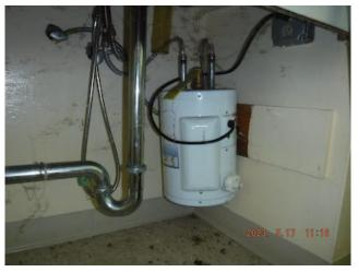
There was no hot water at the time of our inspection. The water heater was plugged into an operating electrical outlet and so is likely to have failed.
