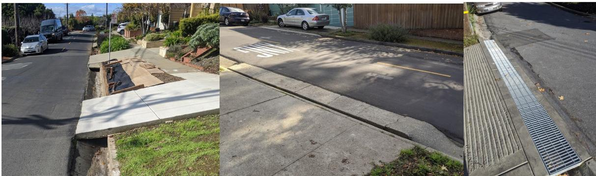
Figure 8: Three variations of driveway gutter crossings: Hard edge (left), smooth edge (center), and metal grate (right).
