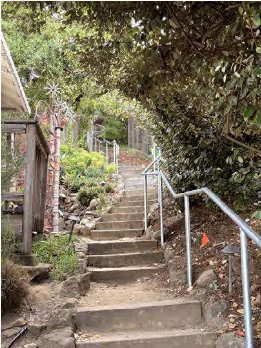
Beloit lower - After with Handrail
