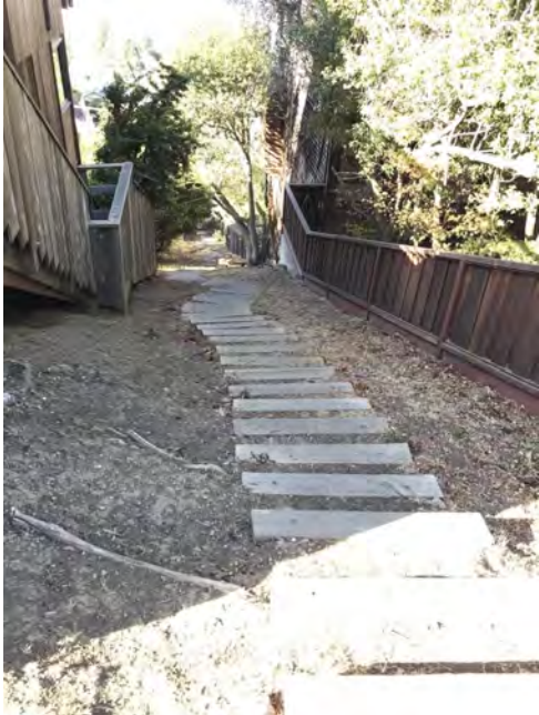
Beloit Lower - Before Handrail
