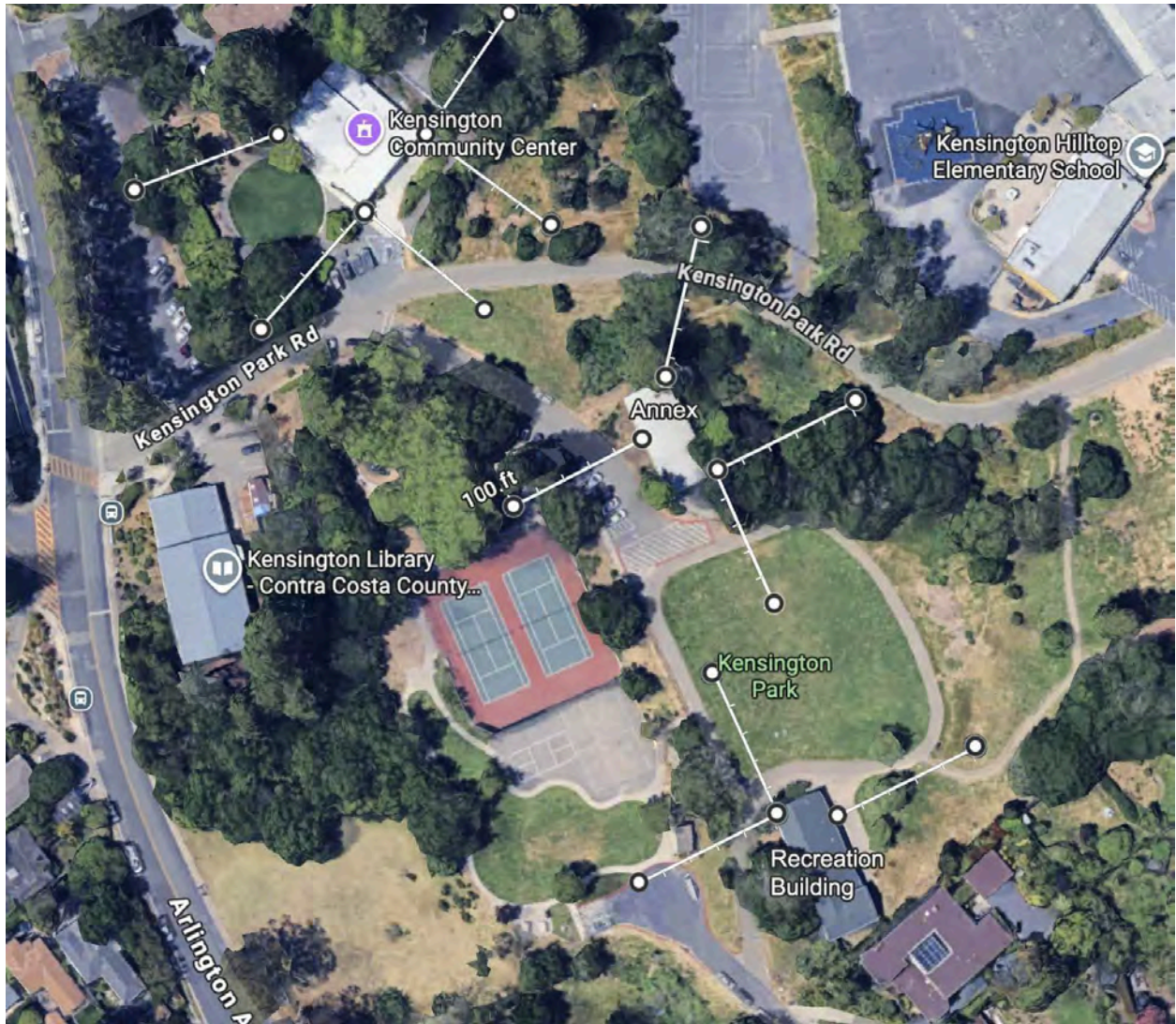
Photo: Aerial view of Kensington Park with 100' defensible space zones marked in white for each building in the assessment.
