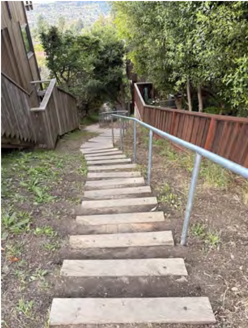
Beloit Lower - After with Handrail
