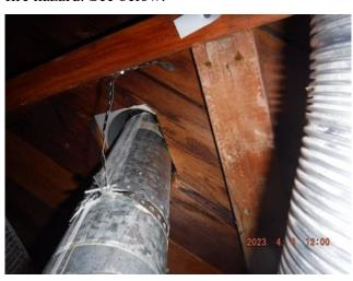
We recommend adequate vent pipe clearance be provided. Double-wall vent pipes need at least 1-inch clearance from combustibles.
