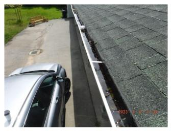
We recommend the gutters be cleaned and re-examined, and modified as needed to drain freely. Rain gutters should be cleared periodically as part of routine maintenance.
