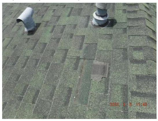
There are several exposed fasteners. With time exposed fasteners will rust and loosen and may cause leakage.
