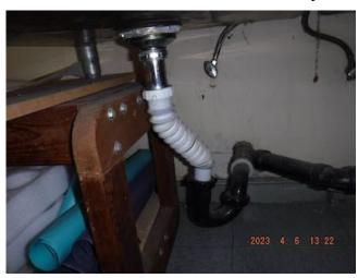
Corrugated drainage connectors are often installed by non-professionals to form drain traps or other drainage connections. These materials do not have smooth interior waterways and collect sludge. They are not approved and should be replaced with conventional drainage fittings and materials.
