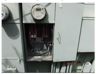
There is both a breaker main panel and a fuse main panel at the left exterior. Fuses in the latter panel are used for high voltage protection, as opposed the more outdated fuses of panels from the 1940 and earlier. The use of fuses (T type 200 amp shown below) in this case is not a concern for us, though more modern equipment will generally use solely breakers and add convenience.
