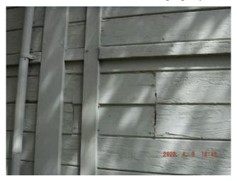
Low voltage electrical equipment is mounted on the left-hand side of the building using a plywood panel which has become loose from the siding.
