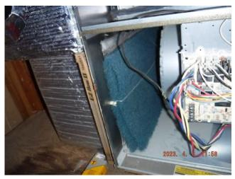
Air filters prevent the accumulation of dust and dirt on the blower fan blades which can significantly reduce efficiency. Air filters should be checked monthly and changed or cleaned, depending on type, as necessary. A clogged air filter can lead to reduced air flow over a furnace heat exchanger, resulting in premature heat exchanger cracking or failure.
