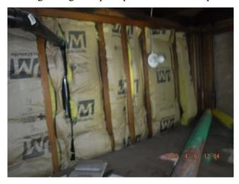
Inverted vapor barriers can constitute a fire hazard. A warning to this effect is typically found on the insulation vapor barrier. The vapor barrier should be placed against a solid backing, toward the interior of the dwelling and should never be visible from the crawlspace or the attic. In humid environments, this inversion can also cause the accrual of condensation and can damage framing. We recommend vapor barriers be properly placed.
