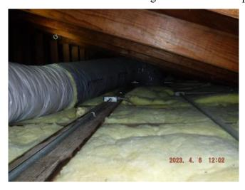
The insulation in the attic vestibules near the furnace has been installed reversed with the paper backing facing the open space. See an example below.
